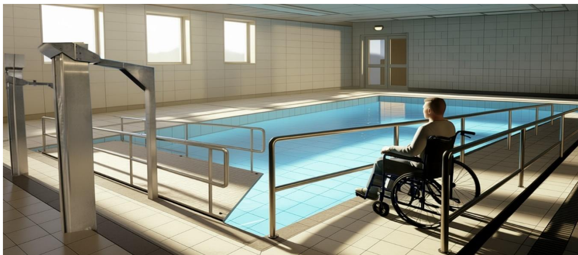
Fig. 2. Main pool equipped with a properly inclined ramp and a Reval-type access platform 1
