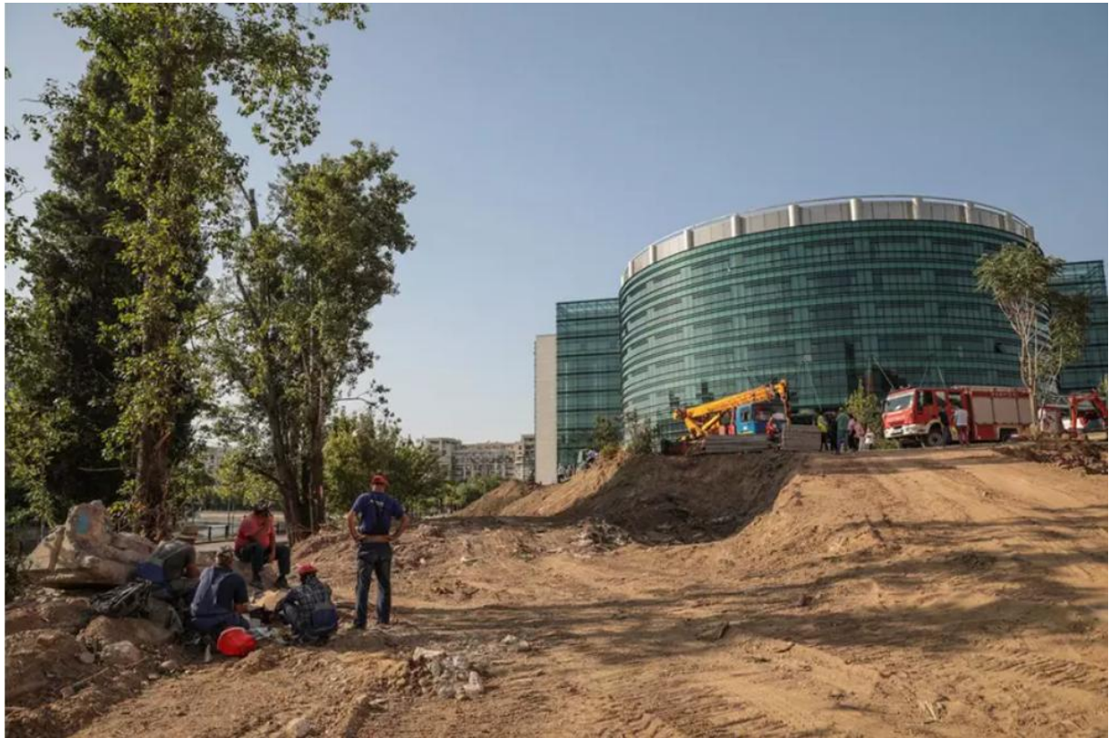
Image 1. The construction site where the accident occurred
