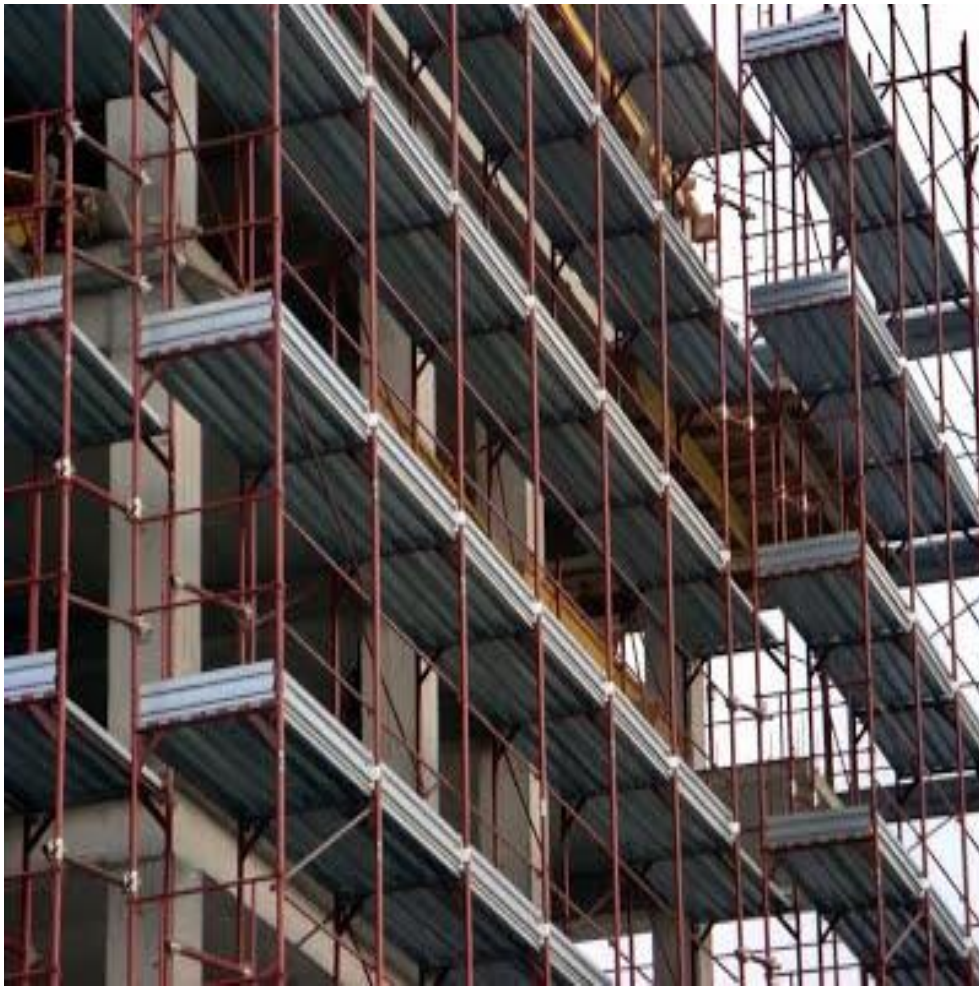
Fig.7. Schela de fatada complete
