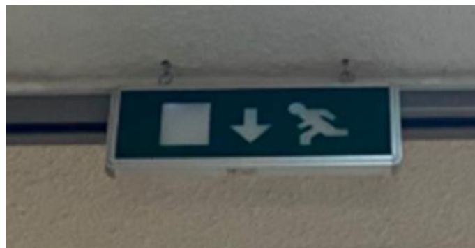
Fig. 8. Light box for highlighting the escape path
