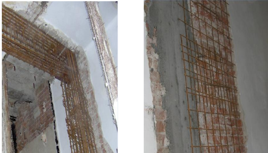
Fig. 4. Reinforcement of the consolidation framework
