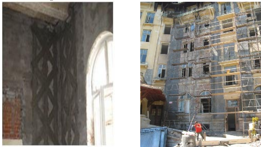
Fig. 5. Strengthening masonry screeds with carbon fibers
